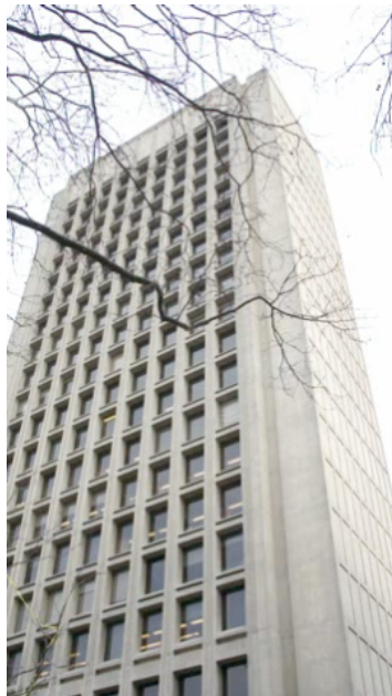
Buildings swaying in wind
