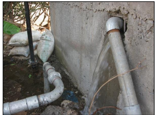
Figure 19: Water overflow from Gudvanwadi sump
