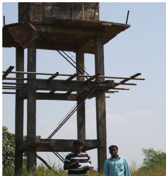
Fig Overhead Tank in Musalepada
