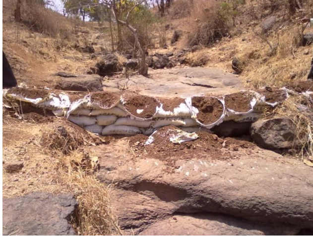
Figure 4.8: Vanrai Bandhara in Washala, Mokhada
