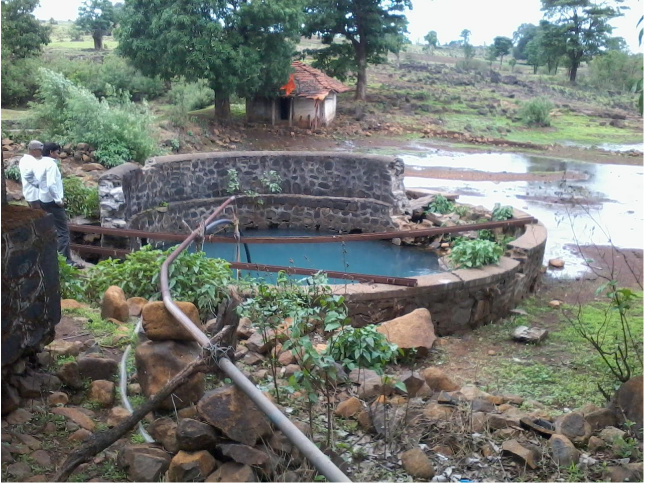
Figure 14 - Suryamal Piped Water Scheme
