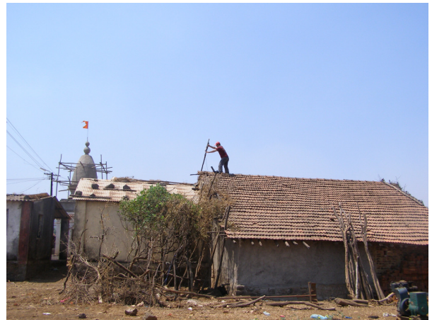
Figure 1: Deployment at Ahupe, setting up antenna for an 802.15.4 node
