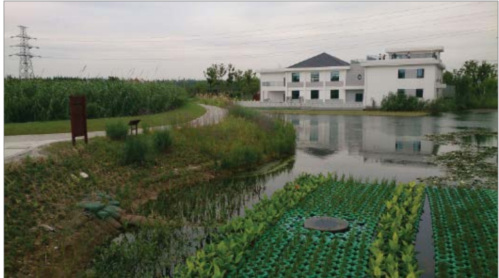
..... Picture 7.4: Constructed wetland in the campus of Indian Agricultural Research Institute, Delhi
