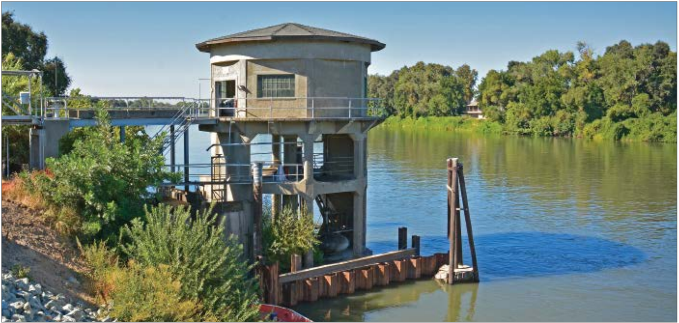
Picture 2.2: River intake structure
