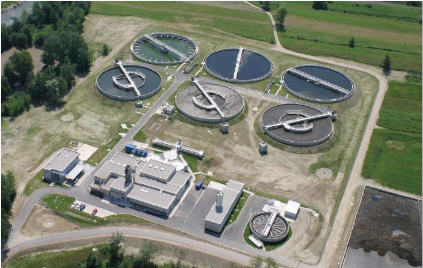
Picture 7.1: A sewage treatment plant
