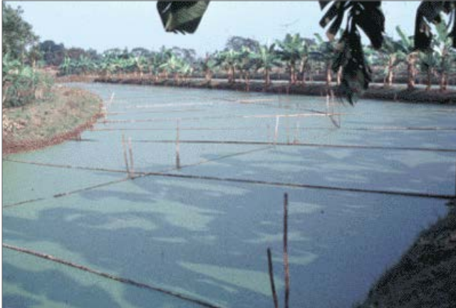
..... Picture 7.3: A duckweed based wastewater treatment system at Mirzapur, Bangladesh (Source: UNEP) and Lemna Minor or common duckweed
