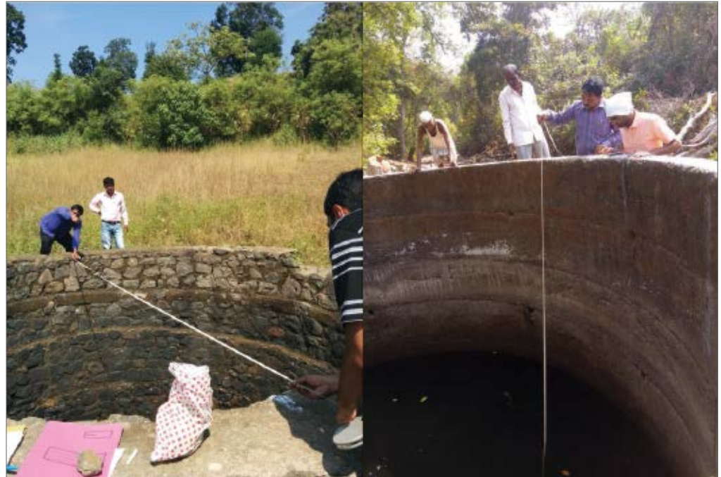
Figure 3B.3: Measuring dimensions of well
