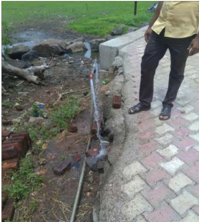
Figure 3C.9: Distribution network laid on ground
