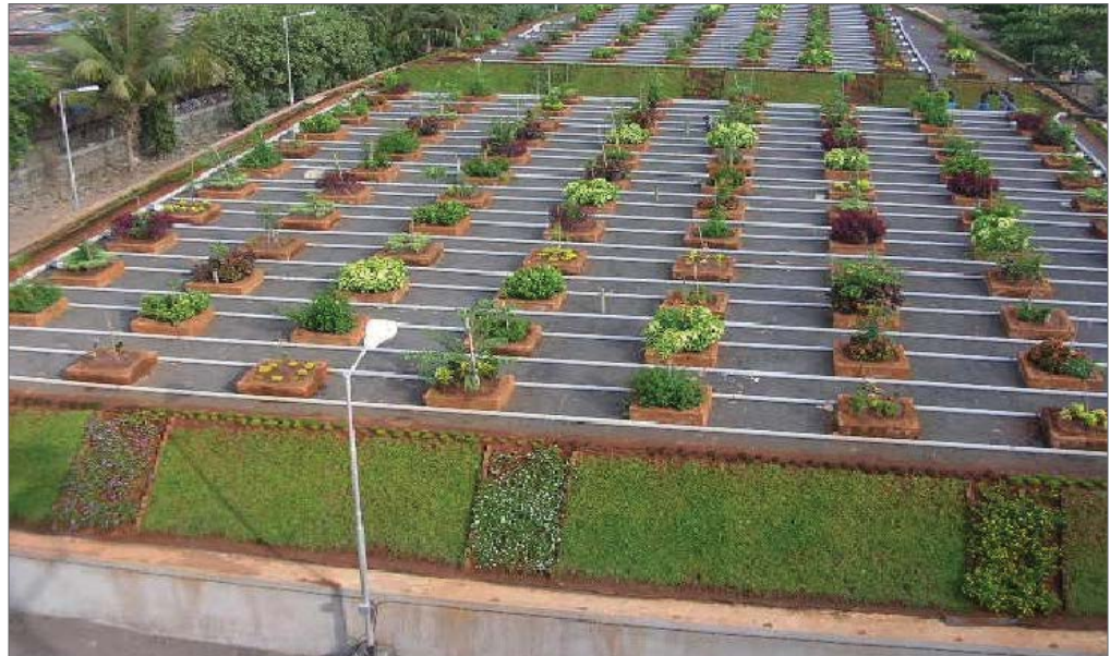
..... Picture 7.2: Soil Bio Technology (SBT) Plant, Mumbai (Implemented by: Mumbai Municipal Corporation & IIT Mumbai)
