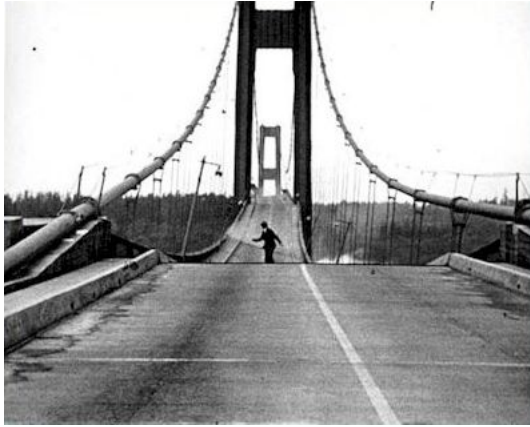
(a) A physicist walking on the antinode line of the standing waves formed on the bridge
