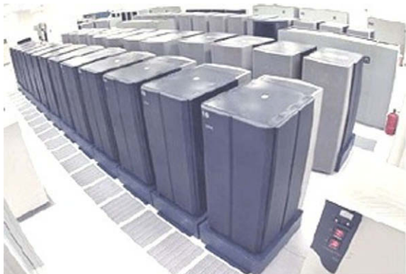
Fig. 1. Physical organization of a data center.
