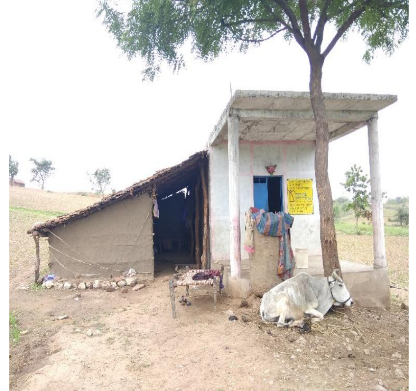
Extension for firewood chulha, made from material of old dismantled House
