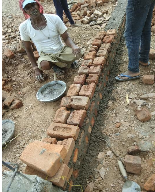
Use of rejected bricks in house construction
