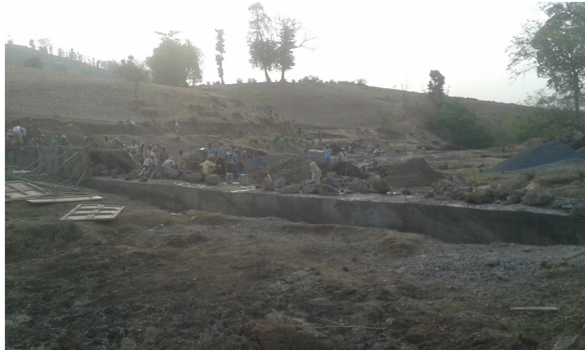
Big boulders in ongoing CNB in Raitale (Jawhar)
