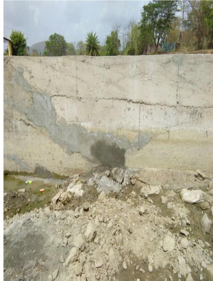
The hole was later patched by the department
