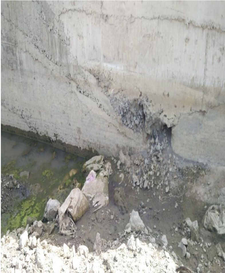
Concrete has come out and reinforcement is visible
