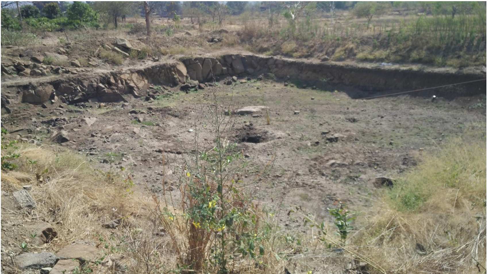
Galtare farm pond gat no 220: soil eroded from the wall, hard strata
