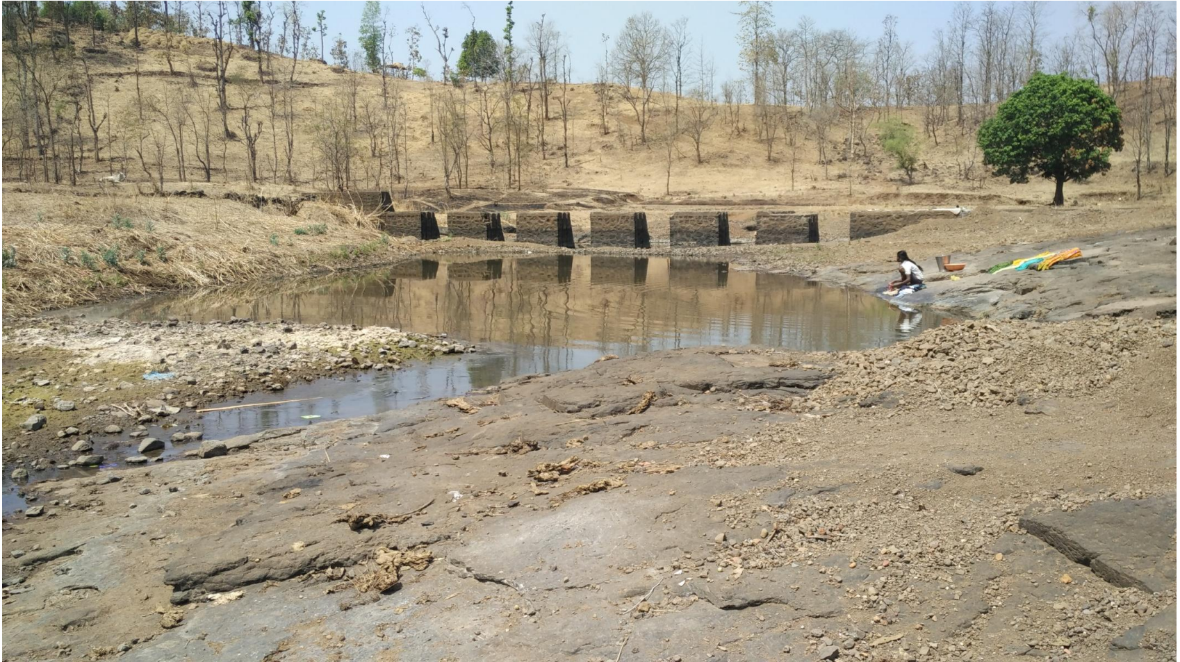
KT bund desilting by forest department in Ujjaini (Wada requires the gates of KT weir
