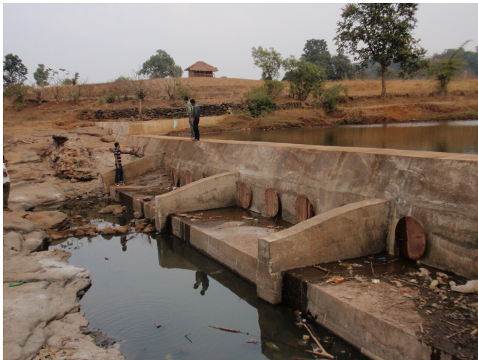
Vented structure at Adoshi.
