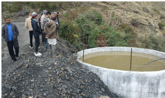
Examine Storage tank
