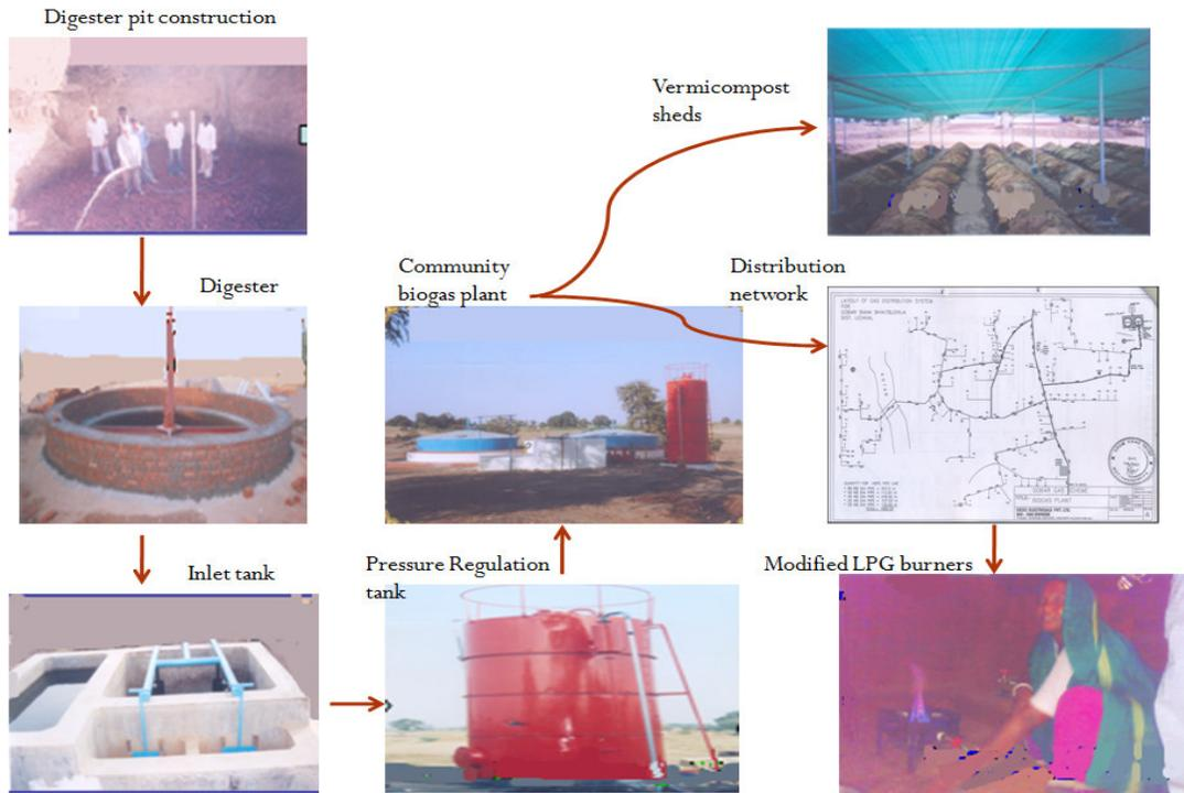
Fig. 2.2 Main stages involved in construction
