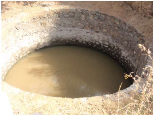
Figure 31 – Photo of incomplete Markatwadi Well 2 (the lining does not even reach ground level).
