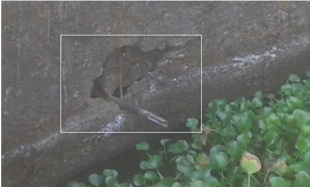
Figure 37 – Damaged well lining
