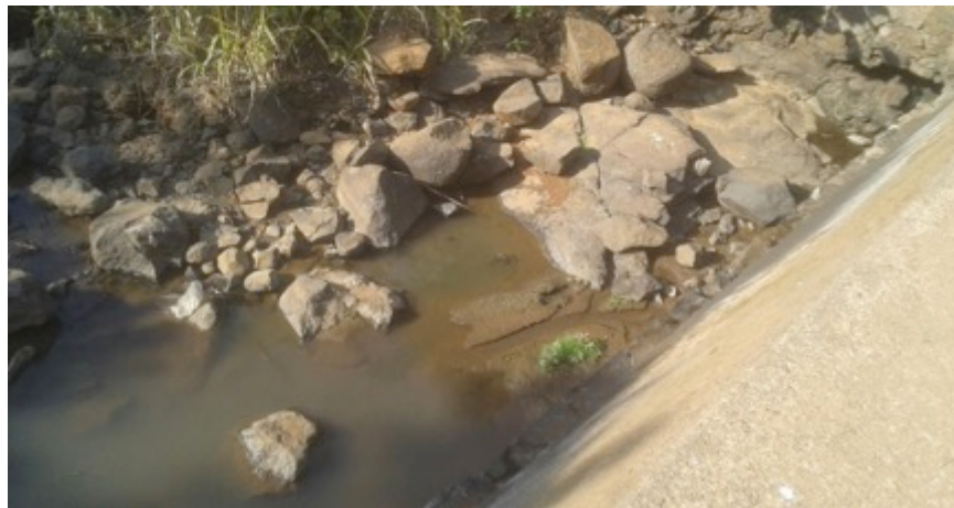
Figure 41 - Leakage from base of Bhojpada bund (downstream).
