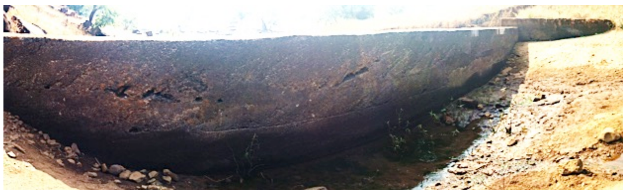
Figure 4 - Photo of the existing bund (upstream) near Kurlod, water is leaking from the base.
