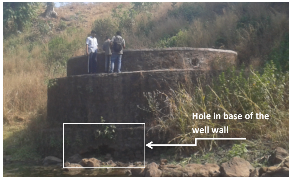
Figure 7 - Photo of Pethechapada's Well 3 showing hole at base of platform.
