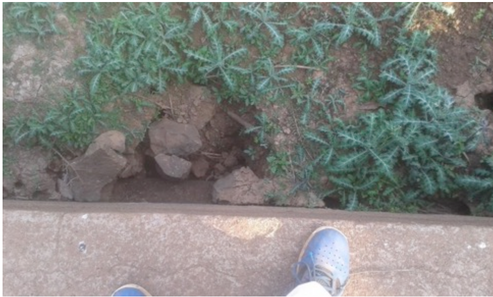
Figure 40 - Photo showing leakage from base of Bhojpada Bund 1 (upstream side).
