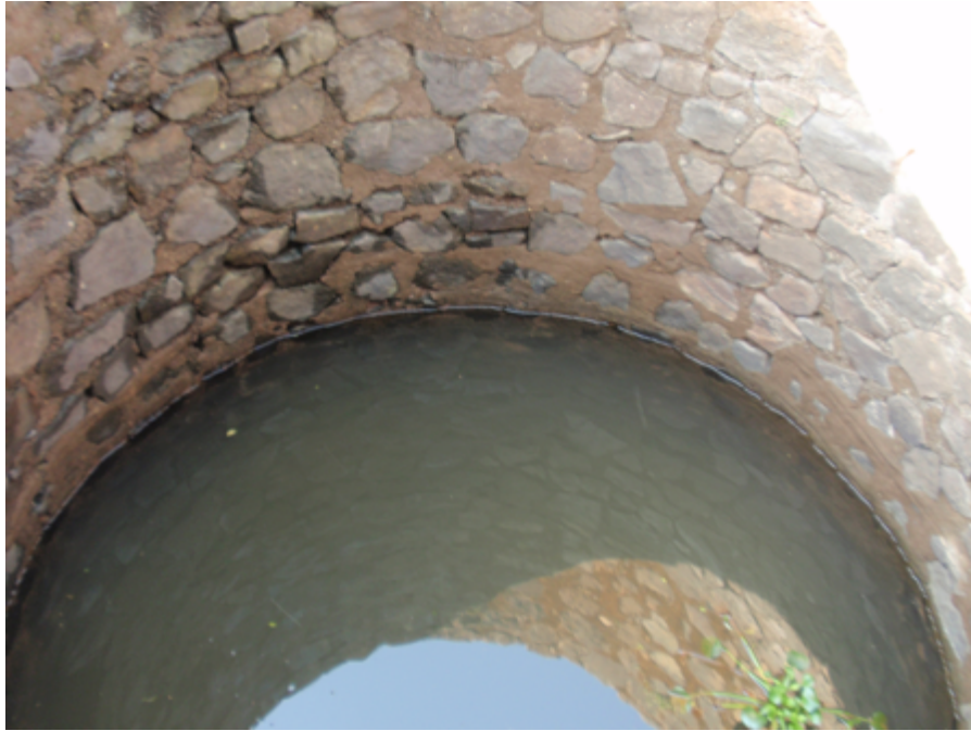
Figure 25 - Photo showing damaged well lining of Kirekirewadi's primary well
