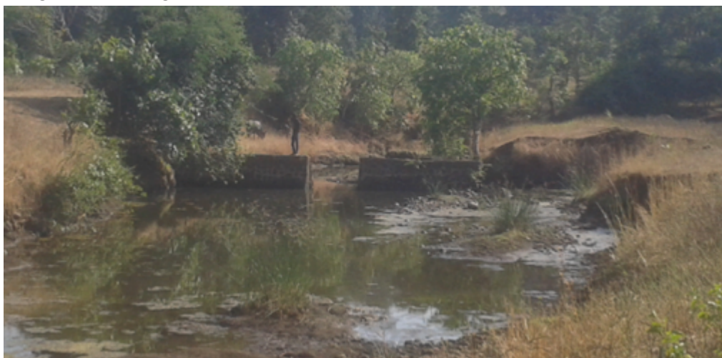
Figure 28 - Photo of Bhelpada's broken bund.
