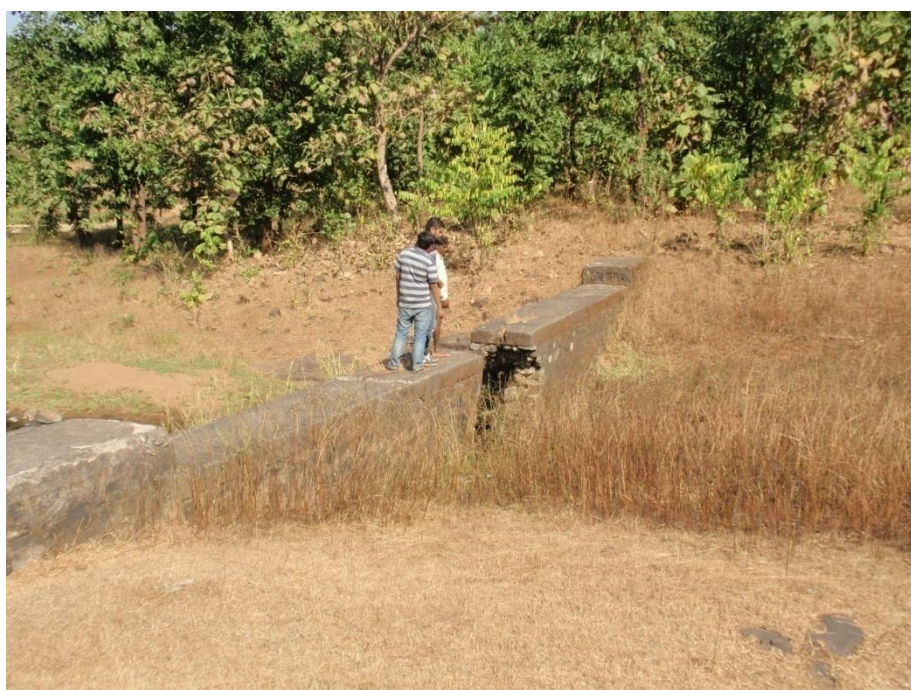
Figure 17 Broken bund (BR1) of Raipada
