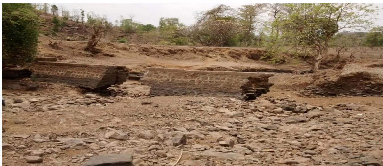
Figure 30 Present condition of Bhelpada Broken bund (BR1)
