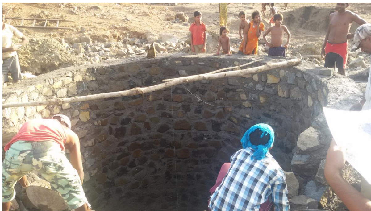
Figure 4 New well construction at Raipada
