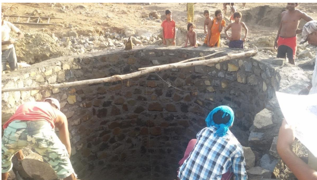
Figure 15 Repair of old primary well (w1) in progress.
