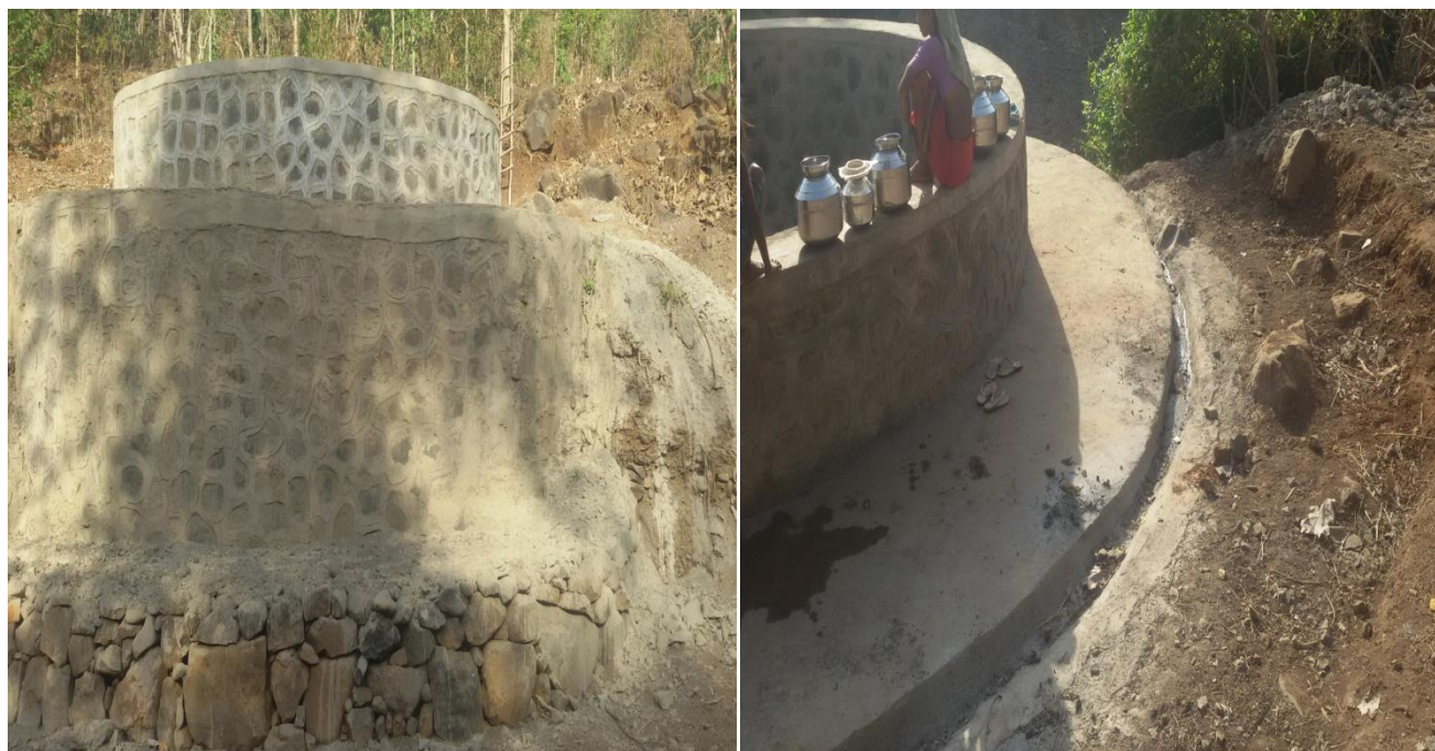
Figure 3 Well lining repair and drainage construction at Kurlod well
