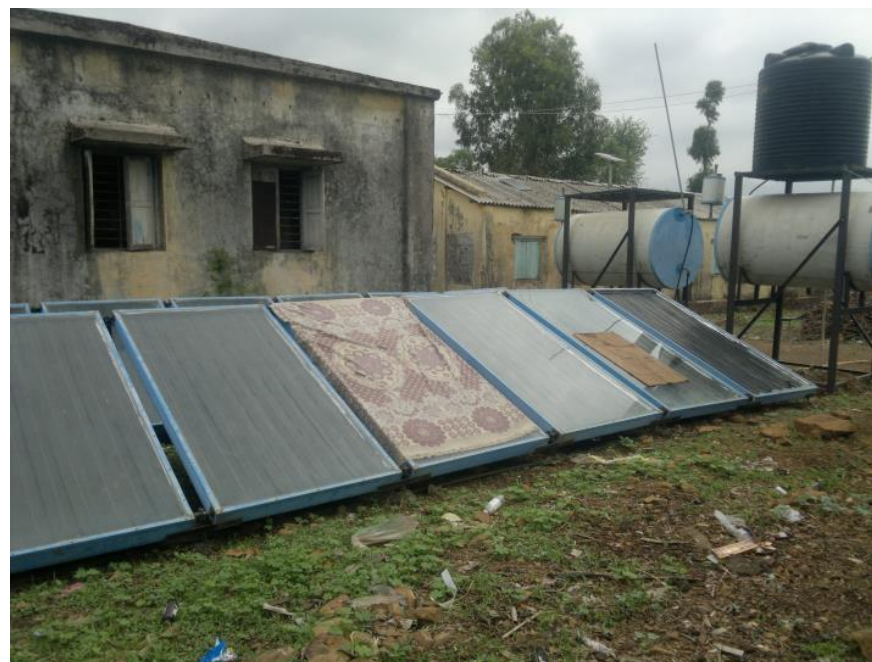
Figure 8-4 : Solar Panels at Ashram Shala
